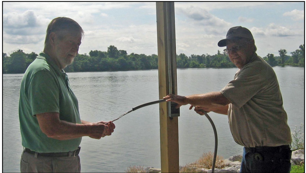
Lodge #572 Veteran's Chairman Steve Schemonia (on left) assists John Burford with installation of new electrical circuits for lighting and power outlets
